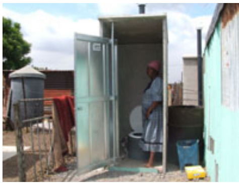
Figure 6 Illustration of a ventilated improved pit latrine.
