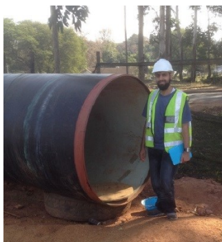
Figure 15 - Photograph of a 1.4m, 400 Mℓ/day pipe at the AD BPT site.
