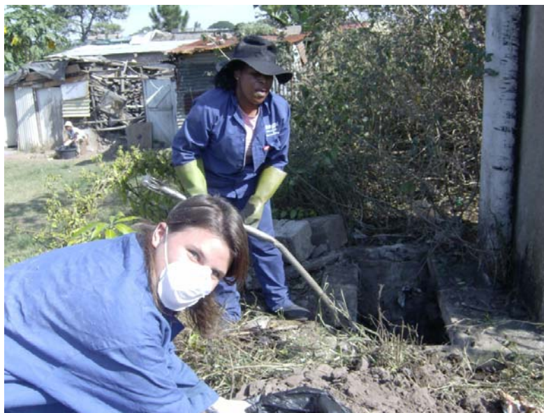
Figure 4.1: VIP emptying and sampling through the back opening
