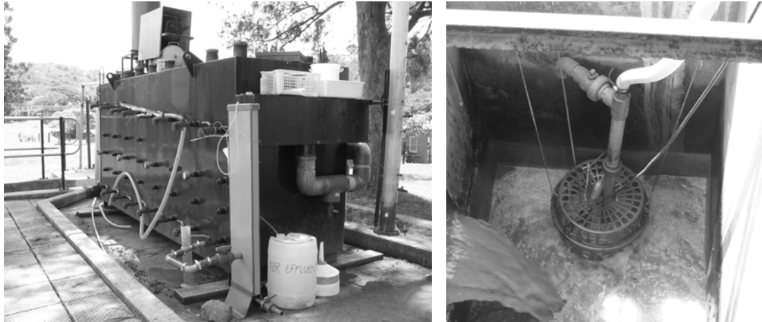
Figure 3.1: Installation of the pilot-scale ABR (3 000 L) at the Kingsburgh WWTP. The outlet end of the pilot ABR showing the membrane unit (Kubota) attached to the last compartment (left); and a laundry basket housing the submersible pump in a wastewater channel, near the feed end of the ABR (right). Taken from Foxon et al. (2005).
