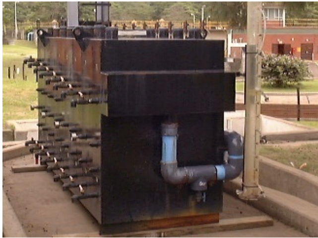
Figure 5.1 Installation of the ABR at Kingsburgh WWTP. The outlet end of the pilot-scale ABR (left); and a laundry basket housing the submersible pump in a wastewater sump near the feed end of the ABR (right)
