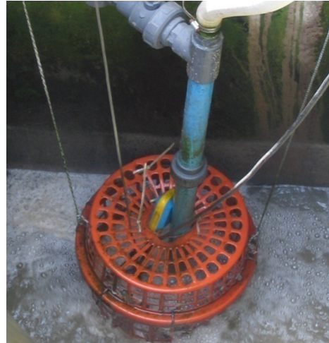
Figure 5.1 Installation of the ABR at Kingsburgh WWTP. The outlet end of the pilot-scale ABR (left); and a laundry basket housing the submersible pump in a wastewater sump near the feed end of the ABR (right)
