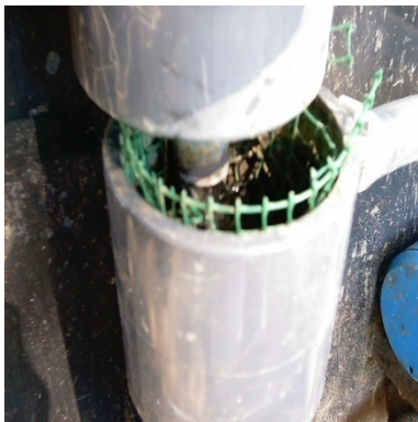
Figure 5.2: Modified outlet of the ABR showing mesh for preventing coarse solids entering the flow meter.
