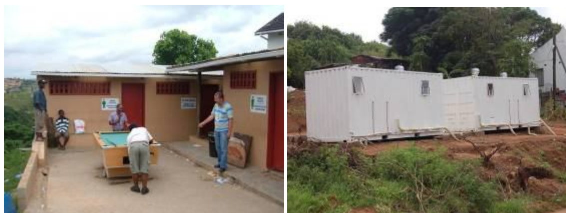
Figure 3: Permanent Ablution Block (Left), Temporary Ablution Block (Right)
