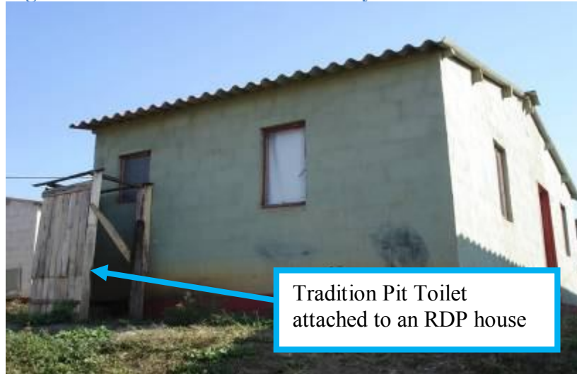
Figure 10: A Pit Latrine next to newly built RDP House in Amawoti-Cuba
