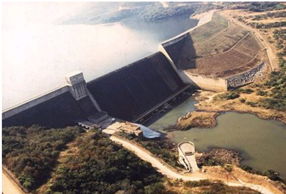
Figure 2-3 Photograph showing the dam wall of Inanda Dam
