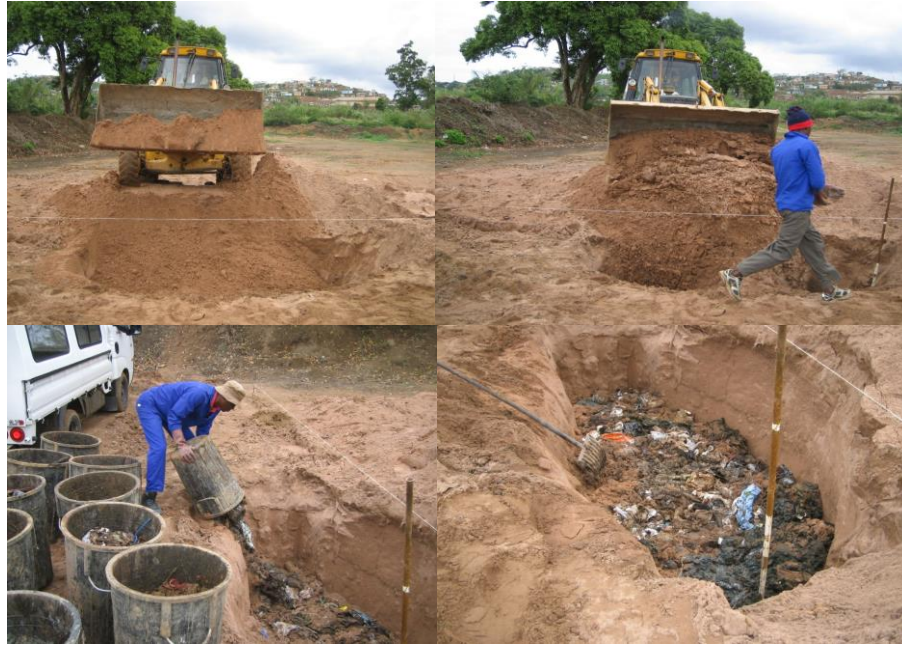
Figure 5.3: Excavation and Sludge burial in Trenches at the Umlazi Site
