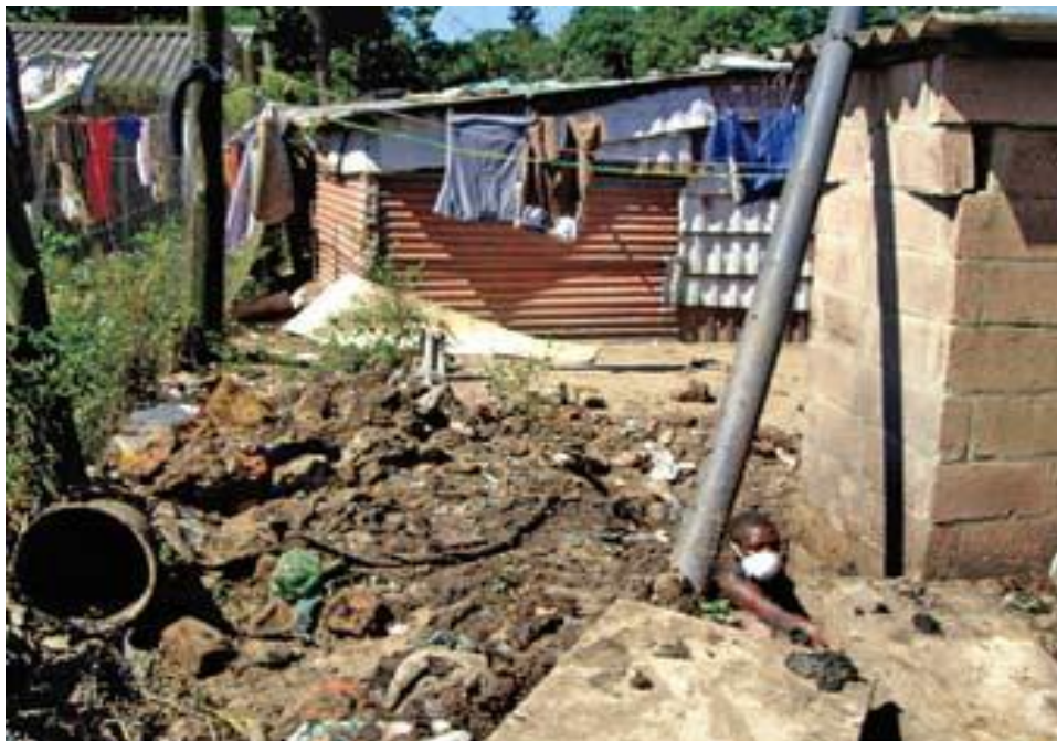
Figure 2.7: Manual pit emptying.
