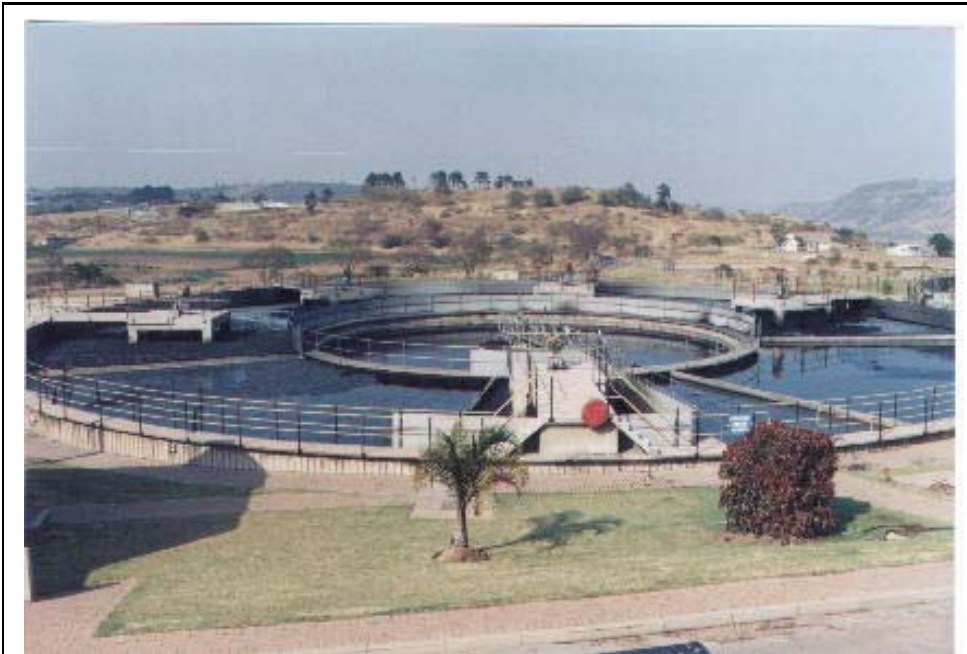
Figure A.2 : A view of one of the 5-stage Bardenpho reactors with the anaerobic and primary anoxic zones to the right of the picture.
