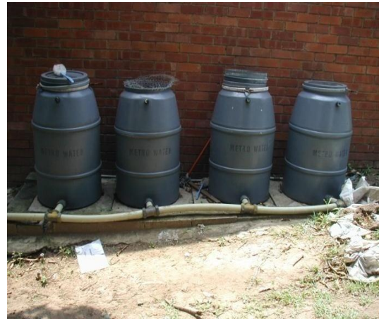
Figure 2.3: Greywater storage tanks at pilot site
