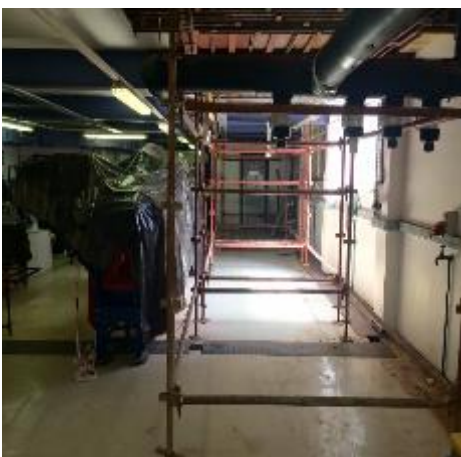
Figure 3: Basement 2 LaDePa region with scaffolding .
