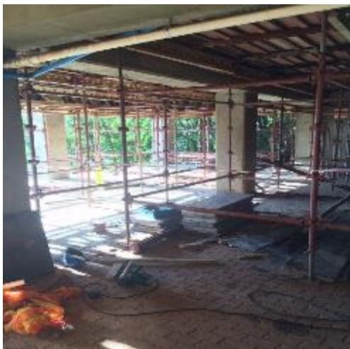
Figure 5: Gas cylinder storage area 1 with scaffolding
