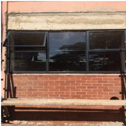
Figure 3: New window installed on the wash basin wall area.
