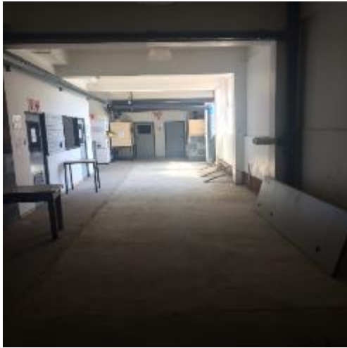
Figure 1: Basement 1 slab finished.
