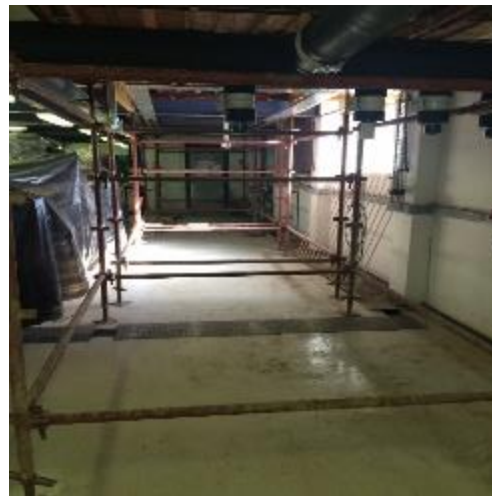
Figure 4: LaDepa region with scafflodng underneath the finished slab.
