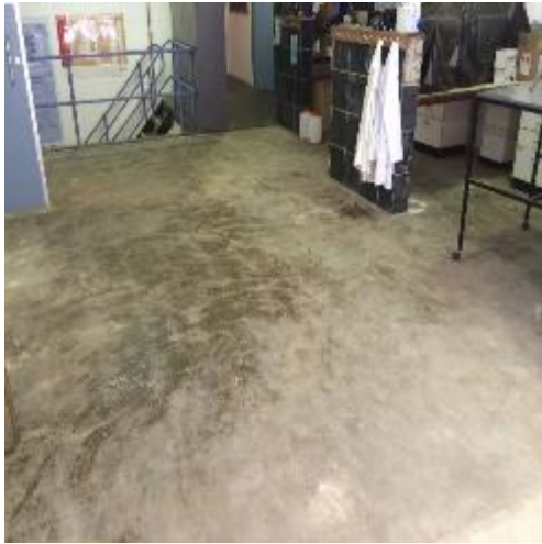
Figure 1: Basement 1 slab finished, tiles completely removed from the whole Basement 1 floor.
