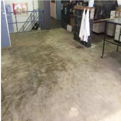
Figure 1: Basement 1 slab finished, tiles completely removed from the floor.
