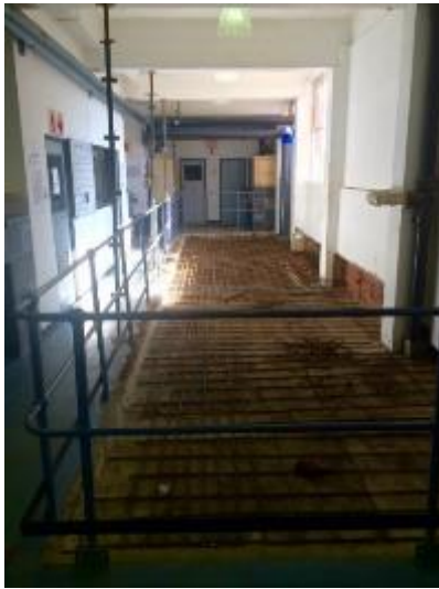
Figure 1: Basement 1 slab foundation with metal reinforcement grid.
