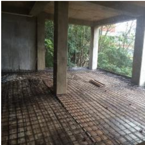
Figure 3: New slab foundation with grid layer (underpinning) View from the office window.
