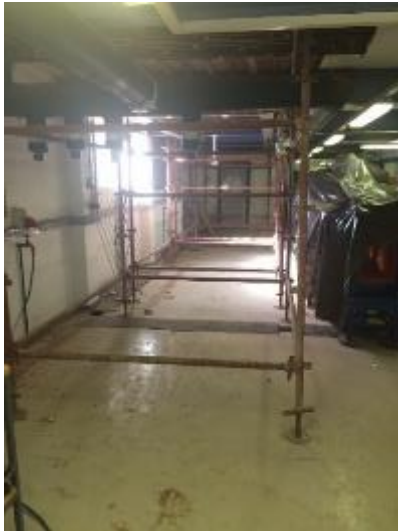
Figure 3: Basement 2 LaDePa region with scaffolding.
