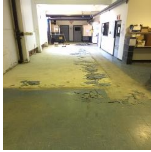
Figure 2: Removal of tiles in basement 1.
