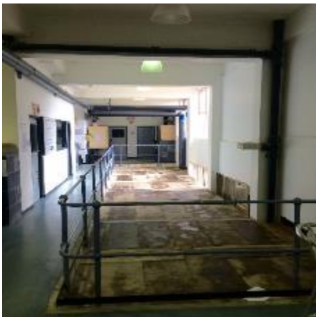
Figure 1: Basement 1 slab foundation.
