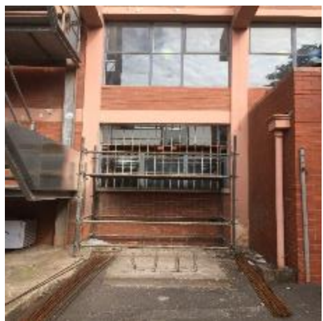
Figure 4: Wash station with hole and scaffolding staging and filters removed.
