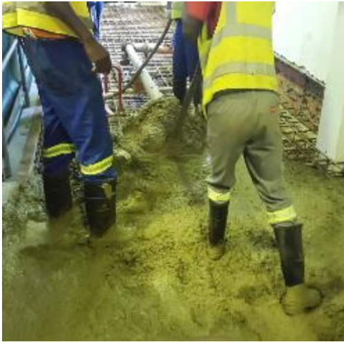
Figure 1: Cementing of Basement 1.
