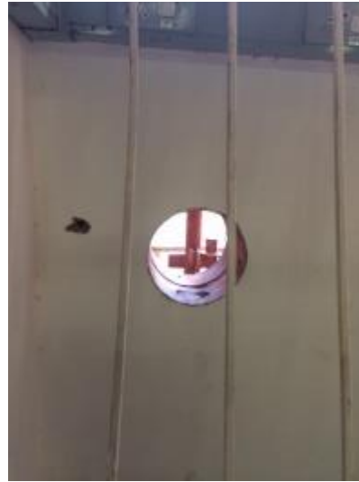
Figure 2: Hole made for the wash station.
