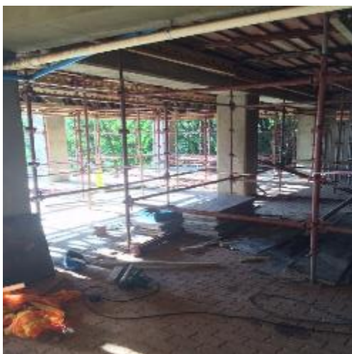
Figure 5: Gas cylinder storage area 1 with scaffolding.
