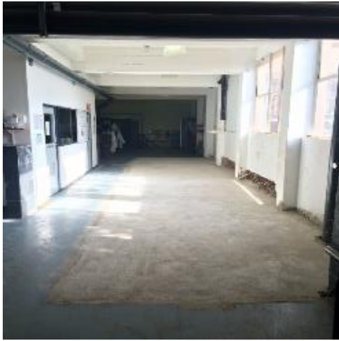
Figure 1: Basement 1 slab finished.
