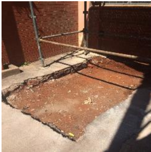
Figure 3: Concrete removed from the wash basin area.
