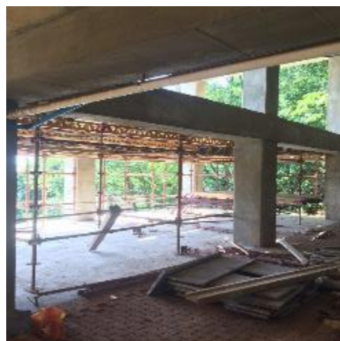
Figure 6: Gas cylinder storage area 1 with concrete foundation and scaffolding.
