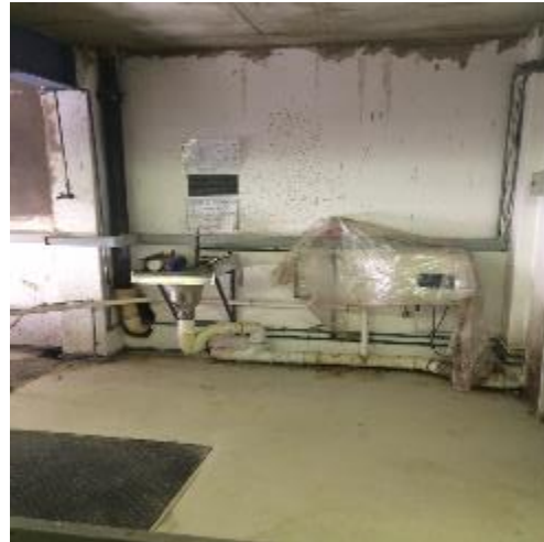
Figure 2: Sink area, scaffolding partially removed, coldroom is accessible.
