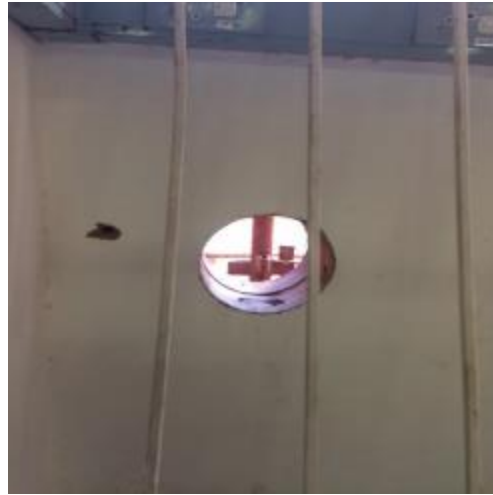
Figure 2: Hole made for wash station.
