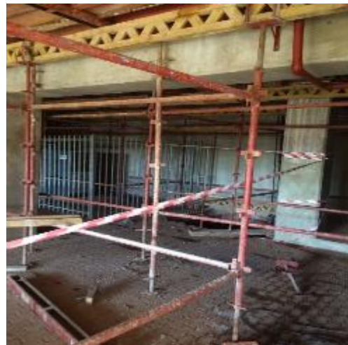
Figure 6: Gas cylinder storage area 2 with scaffolding spanning across area 1 and 2.
