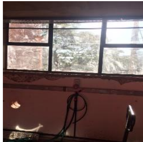
Figure 4: New window. LaDePa region (inside) and wash basin (outside).
