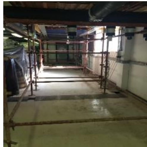
Figure 4: LaDepa region scaffolding underneath the finished slab.
