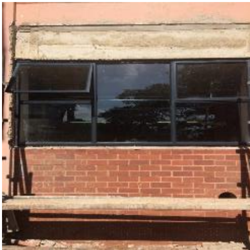
Figure 3: New window installed on the wash basin wall area (outside).
