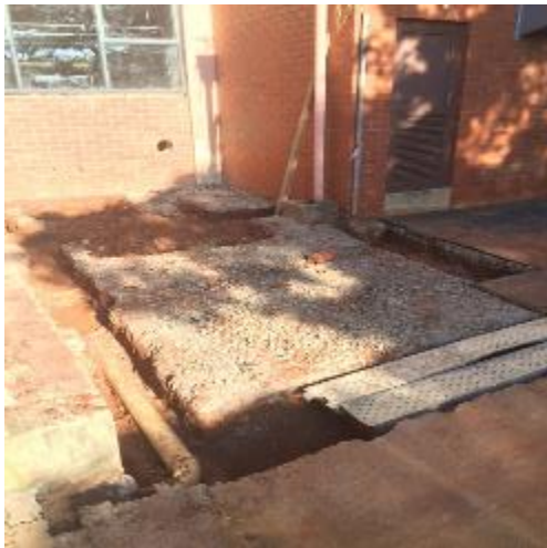
Figure 3: Wash station foundation preparation.
