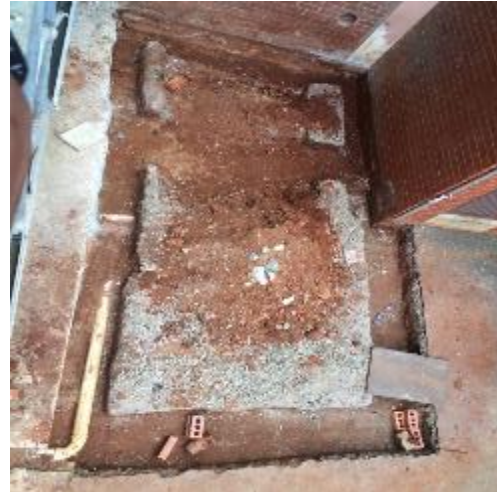
Figure 2: Wash station area, foundation further dug up.
