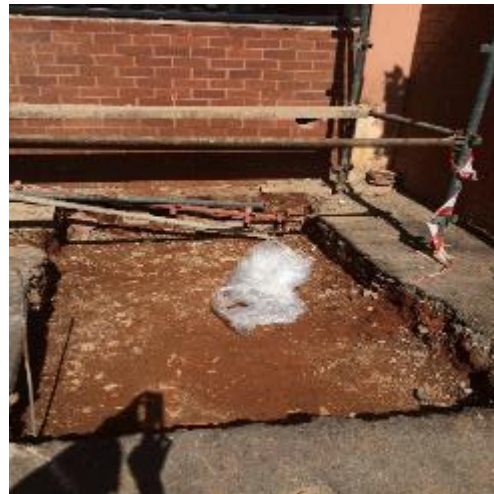
Figure 4: Tar concrete removed from the wash station.
