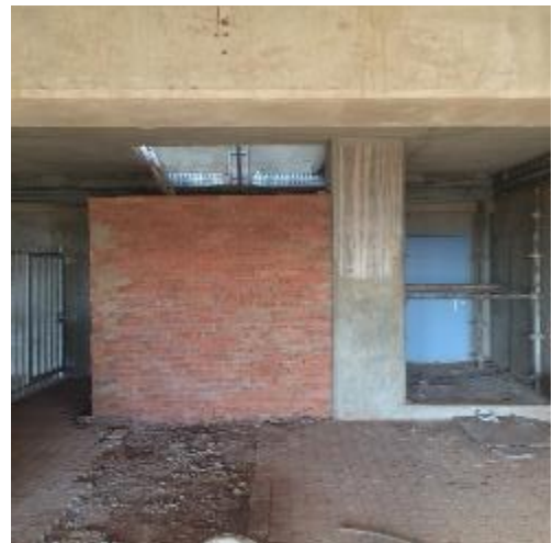
Figure 6: Gas cylinder storage area 2.
