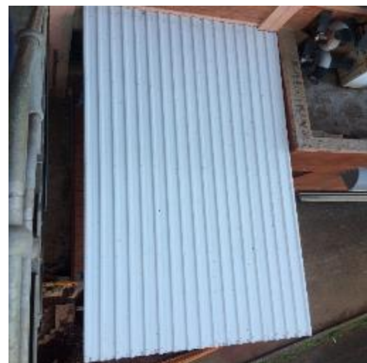
Figure 6: Gas cylinder storage area 2.
