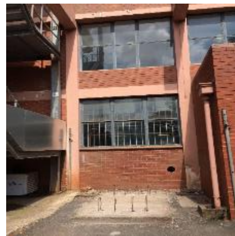
Figure 4: Wash station with drilled hole and filters removed.
