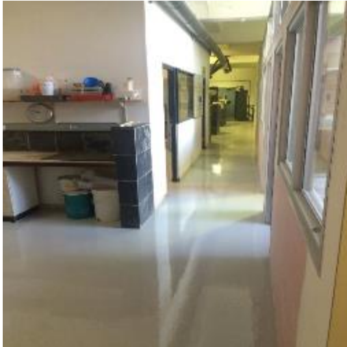
Figure 1: Laboratory Floors refurbished with epoxy coating.
