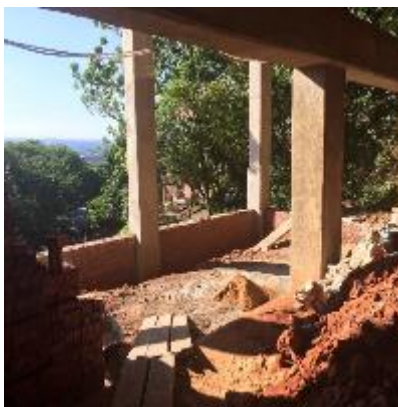
Figure 5: Gas cylinder storage area 1.
