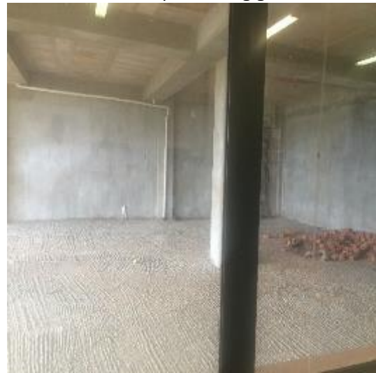
Figure 2: Wash basin foundation, covered with cement and protruding grid.
