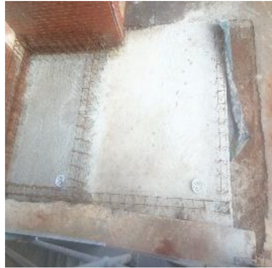
Figure 2: Wash basin foundation, covered with cement and protruding grid.
