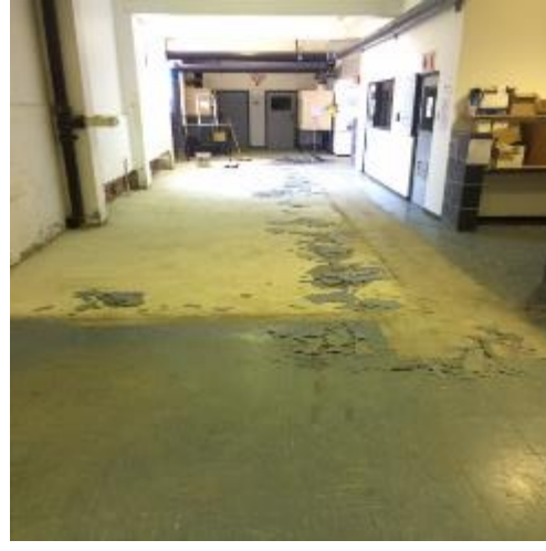
Figure 2: Removal of tiles in basement 1.
