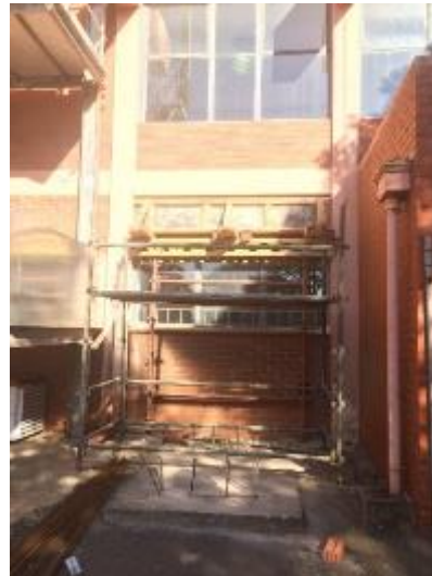
Figure 4: Wash station with hole and scaffolding staging and filters removed.
