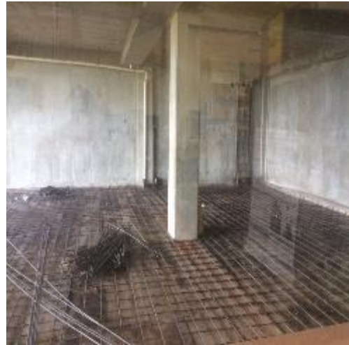
Figure 4: New slab foundation with grid layer (underpinning), above gas cylinder area 2.
