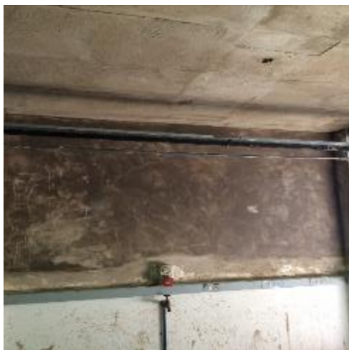
Figure 5: The window that was taken down and cause delays has been sealed.
