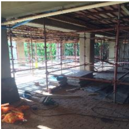
Figure 5: Gas cylinder storage area 1 with scaffolding
