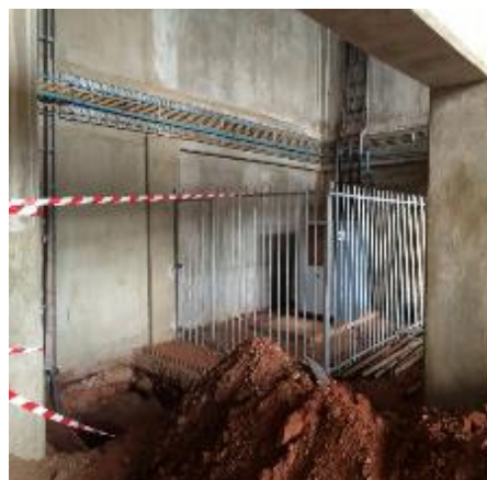
Figure 6: Gas cylinder storage area 2.
