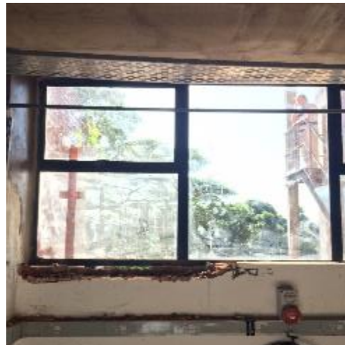
Figure 4: New window installed on the LaDePa area, view from the inside.
