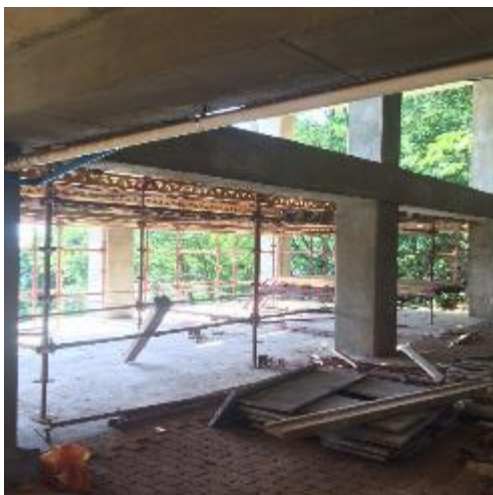
Figure 5: Gas cylinder storage area 1 with concrete foundation and scaffolding.
