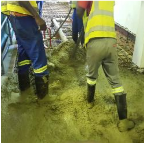
Figure 1: Cementing of Basement 1.
