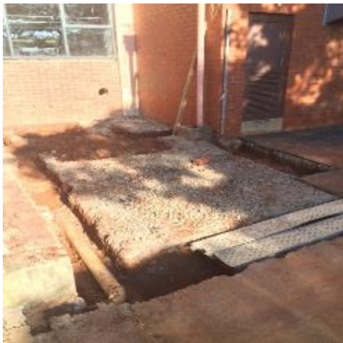
Figure 3: Wash station foundation preparation.
