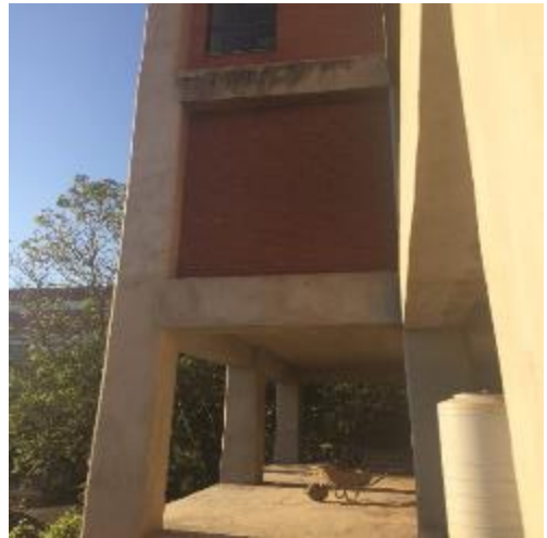
Figure 4: New office area sealed, outside view from PRG office entry.
