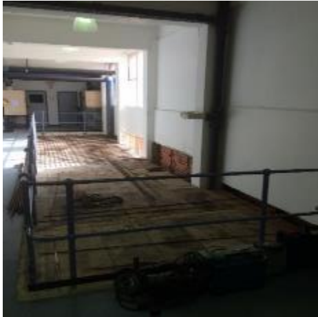
Figure 1: Basement 1 slab foundation with metal reinforcement layer.
