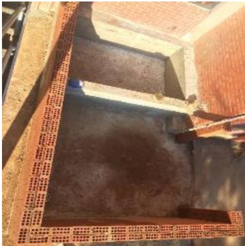
Figure 3: Wash station area.
