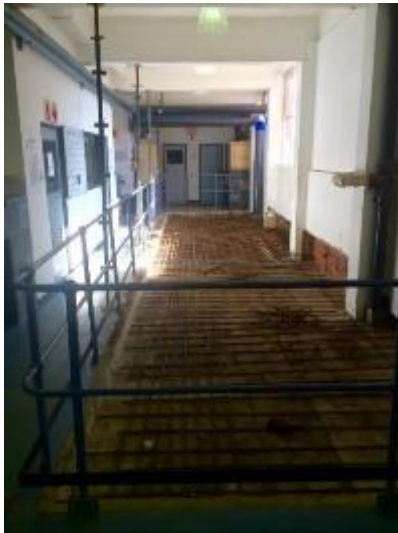
Figure 1: Basement 1 slab foundation with metal reinforcement grid.
