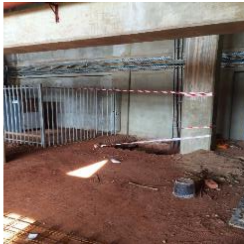
Figure 6: Gas cylinder storage area 2.
