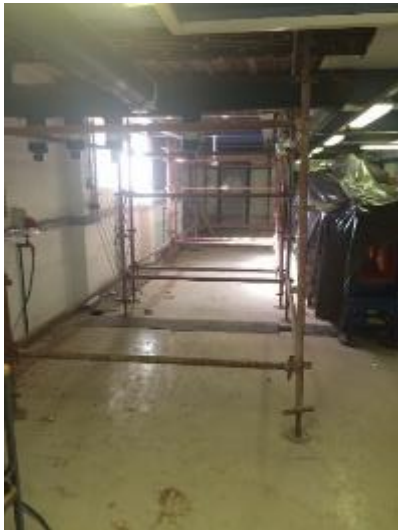
Figure 3: Basement 2 LaDePa region with scaffolding.
