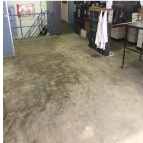
Figure 2: Tiles in Basement 1 completely removed on the floor.
