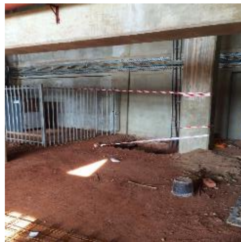
Figure 6: Gas cylinder storage area 2.
