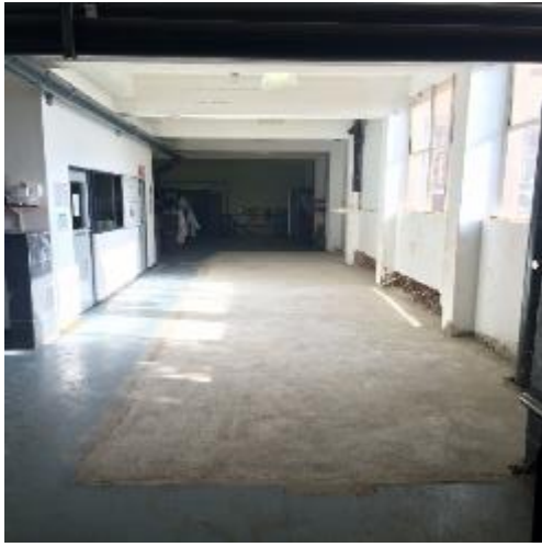
Figure 1: Basement 1 slab finished.
