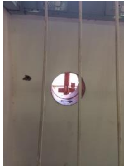
Figure 2: Hole made for the wash station.
