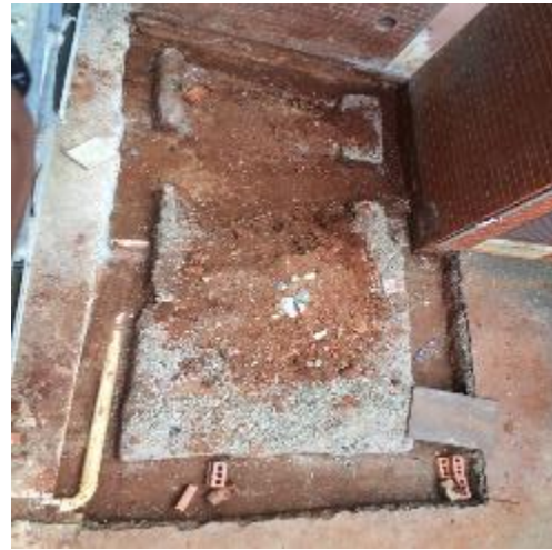
Figure 2: Wash station area, foundation further dug up.
