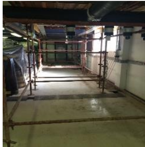
Figure 4: LaDepa region with scaffolding underneath the finished slab.
