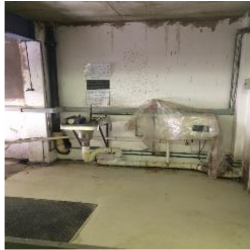
Figure 2: LaDepa region scaffolding partially removed, coldroom is accessible.
