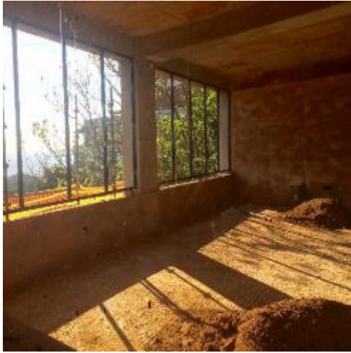
Figure 1: New office area with window frames installed, above gas cylinder storage area 1.
