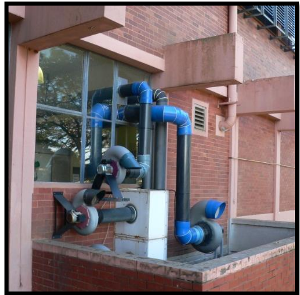
Pathogen filtration Hepa Filters
