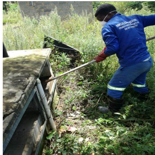
Urine Diversion toilets
