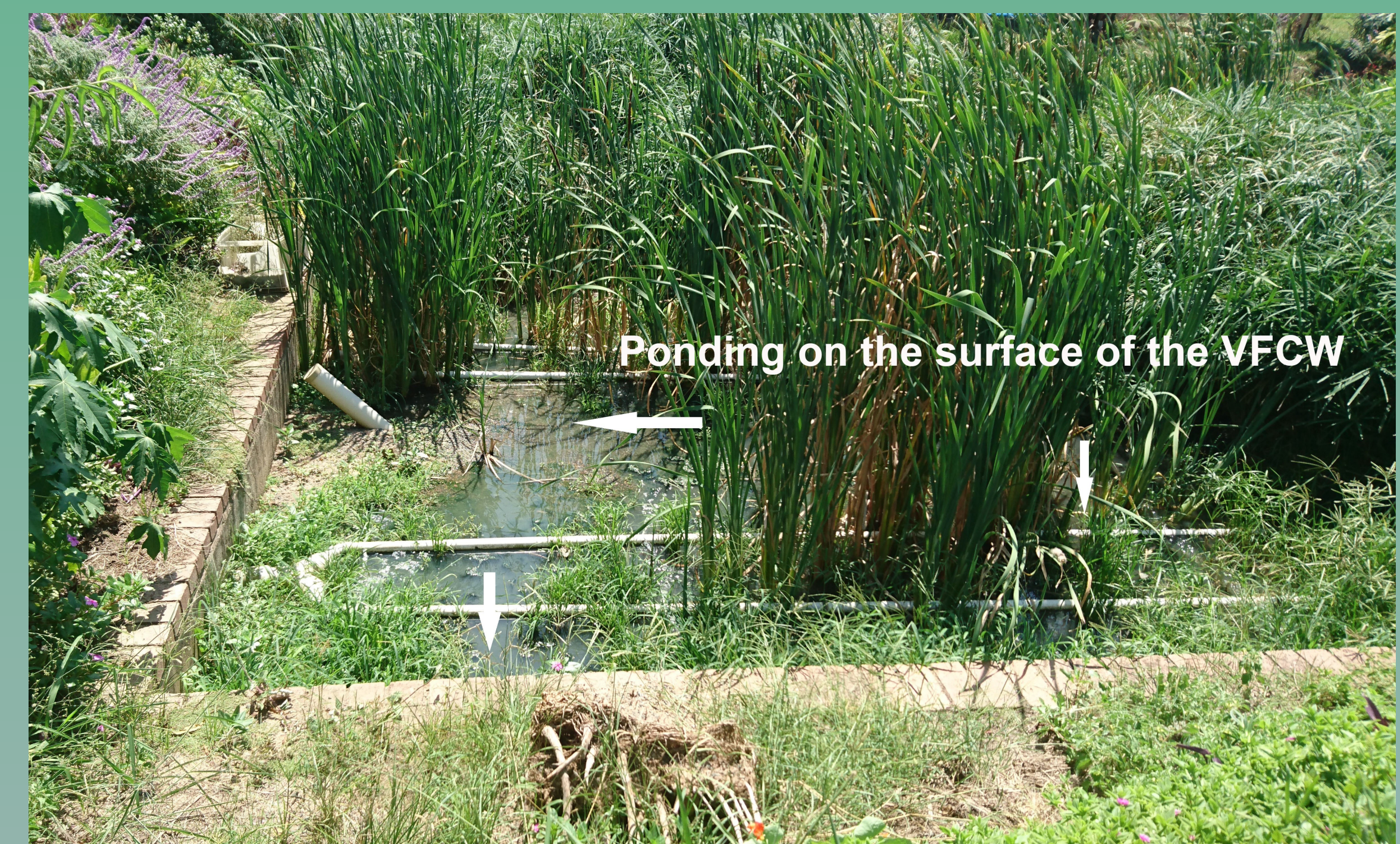
Figure 3: Visible ponding on the surface of the VFCW (taken March 2017)
