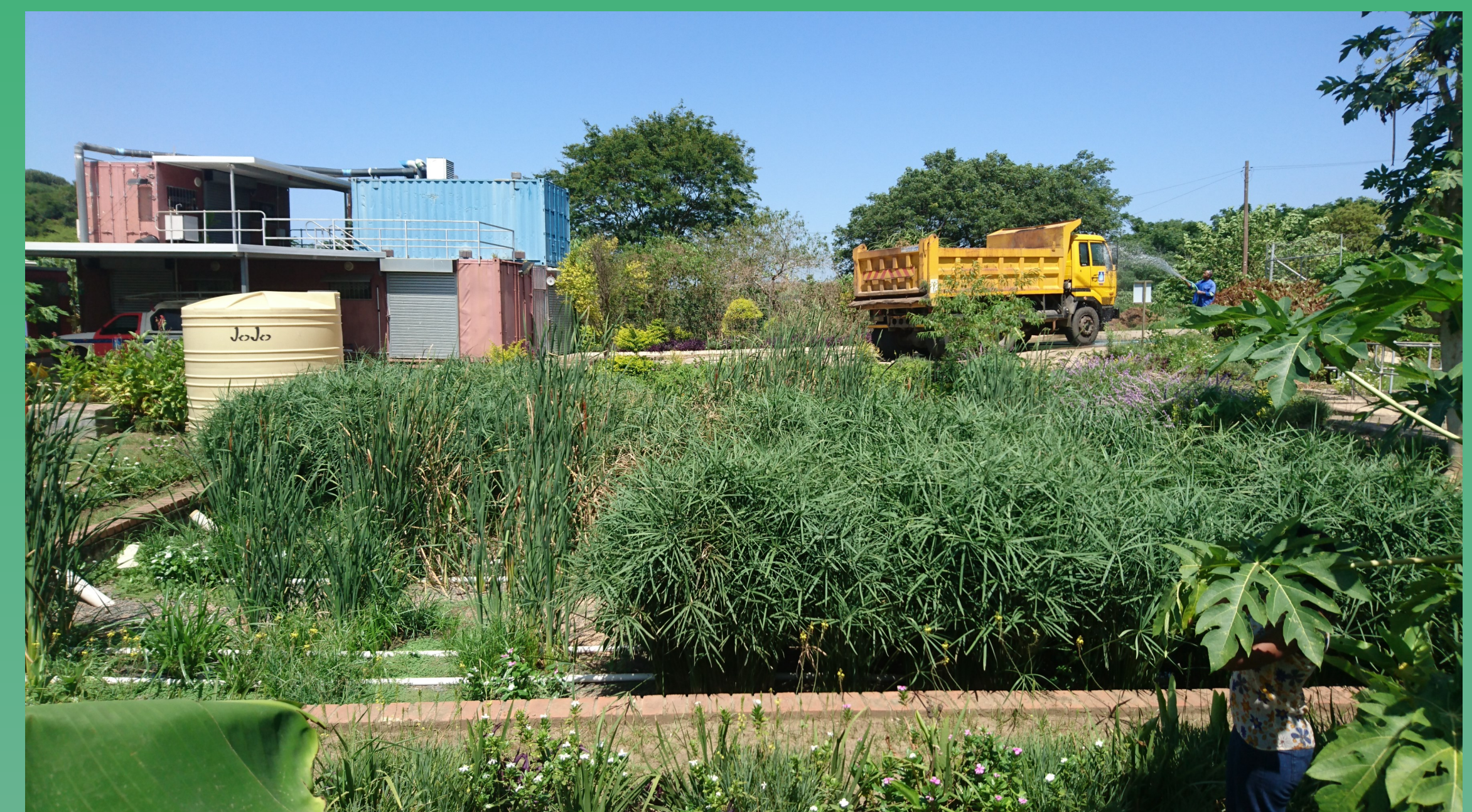
Figure 2: Vertical flow constructed wetlands at the NLM DEWATS (taken December 2016)
