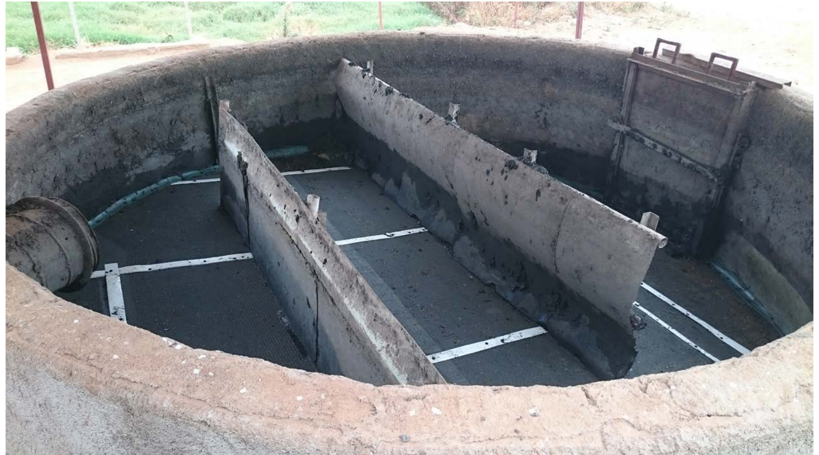
Baffled settling tank for further dewatering
