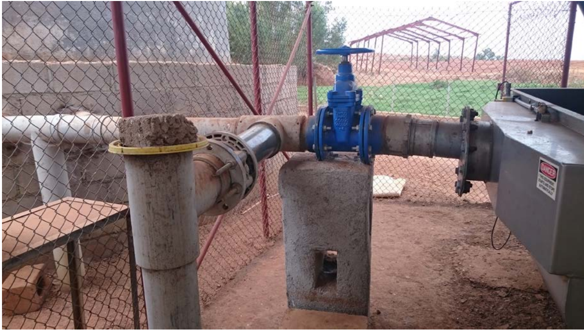
Inlet of faecal sludge into the mechanical dewatering machine
