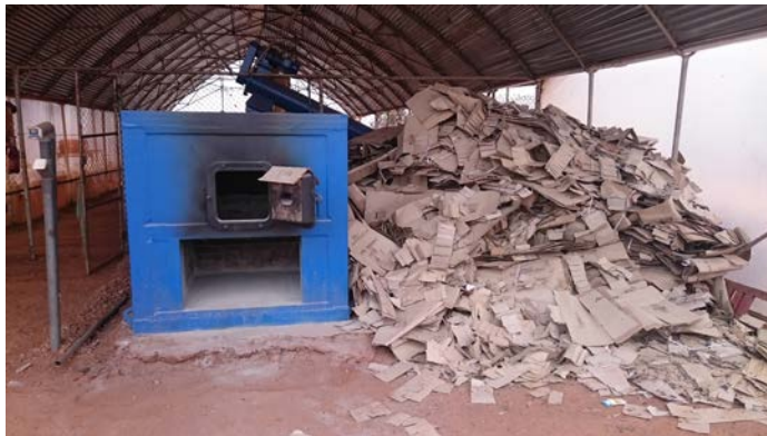
Furnace to provide the heat for drying through cardboard combustion
