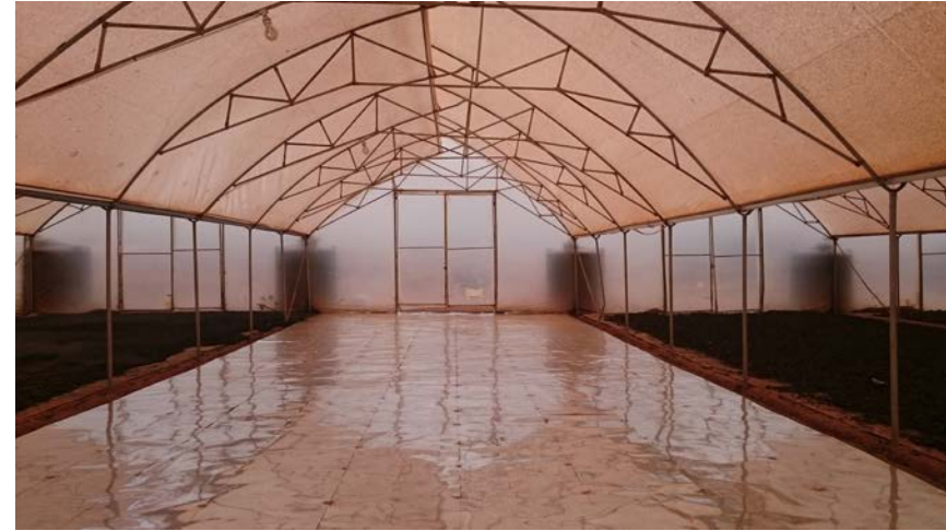
Interior of the greenhouses
