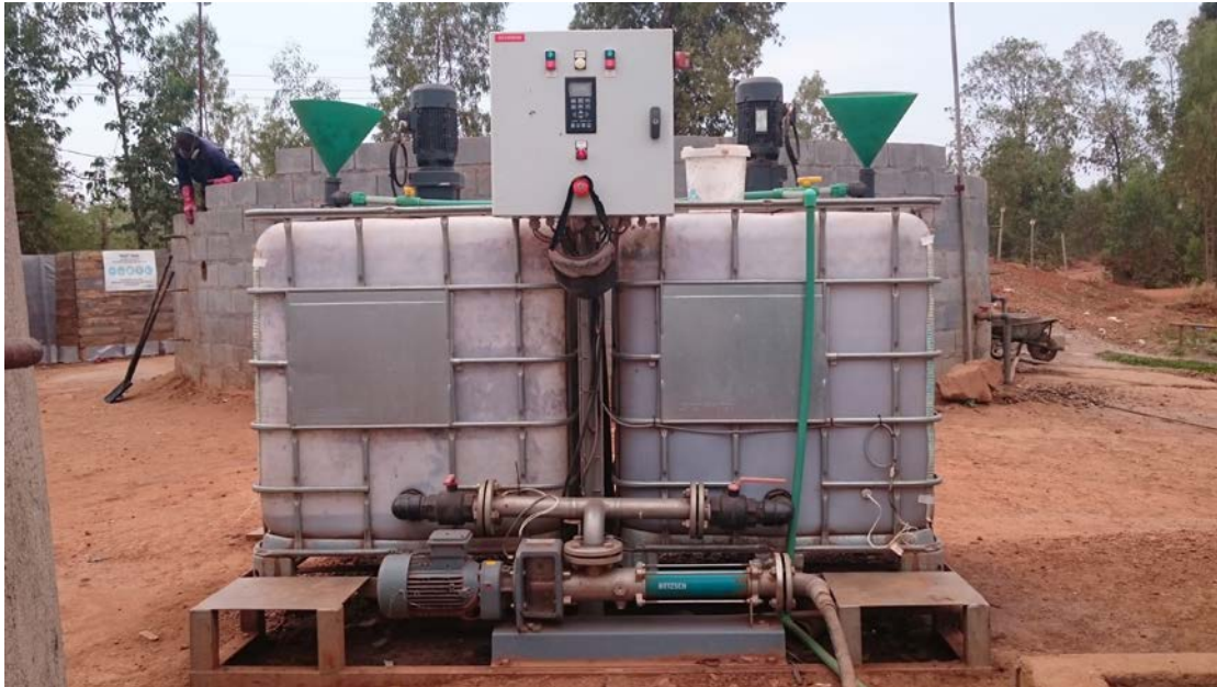
Flocculent solution preparation
