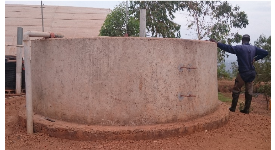
Mixing tank of faecal sludge with flocculent
