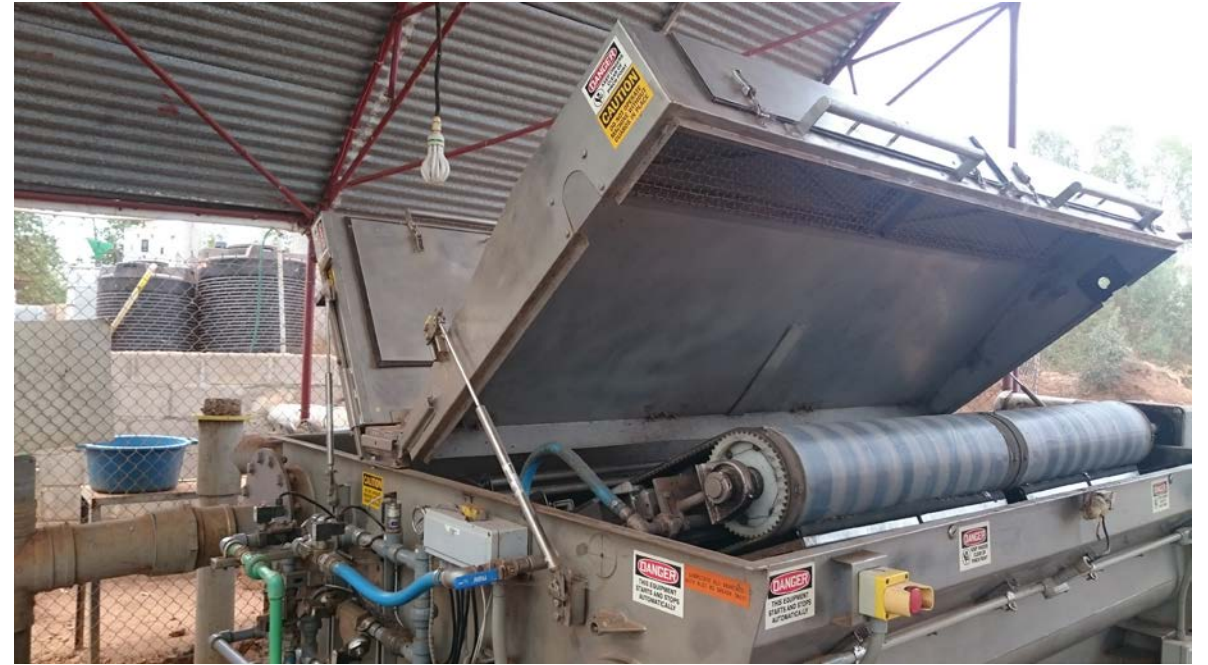
Mechanical dewatering machine
