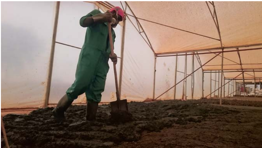
Manual spreading of faecal sludge
