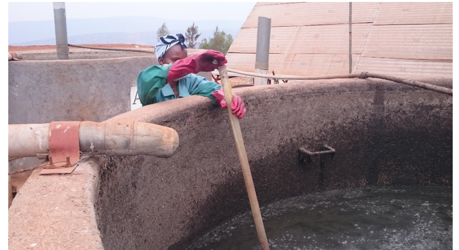
Inlet of flocculent solution and manual mixing
