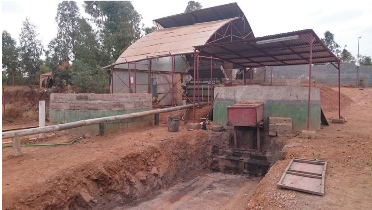
Collection point of dewatered faecal sludge at the outlet of the settling tank
