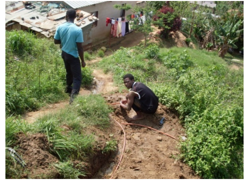
FIG 2: Illegal connections
