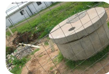
Sewer discharge station
