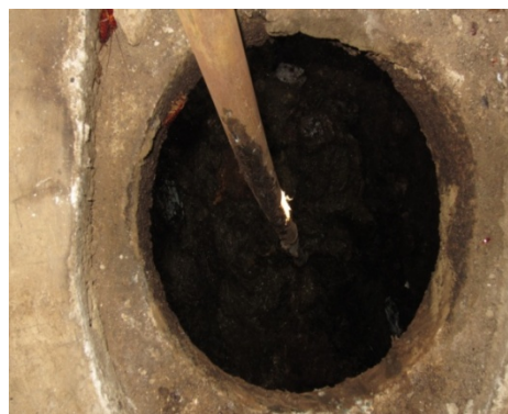
Non-homogeneity of pit latrine contents
