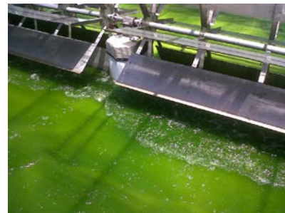
Algae being cultivated in the 300 000 L raceway pond at Kingsburgh wastewater treatment works
