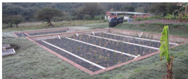
Fig.2: Vertical flow constructed wetland
