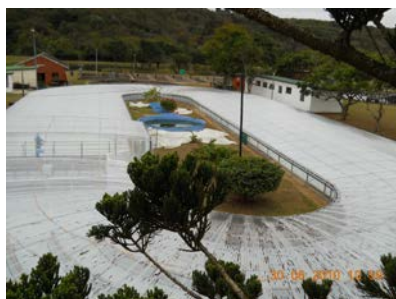
Algae being cultivated in the 300 000 L raceway pond at Kingsburgh wastewater treatment works
