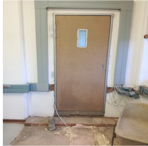
Figure 2: New trunking and step fitted on the meeting lounge side.
