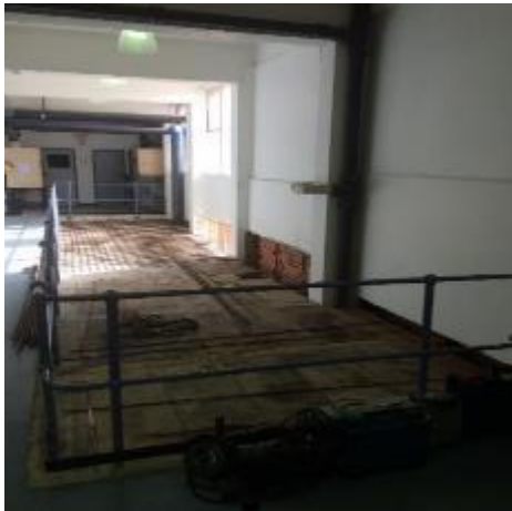
Figure 1: Basement 1 slab foundation with metal reinforcement layer.
