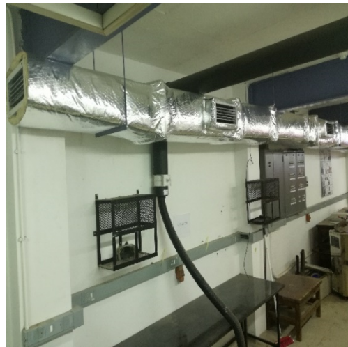
Figure 3.2: Air duct insulation.
