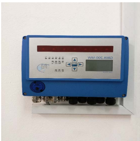
Figure 3.3: Gas leak detectors installed in analytical lab (25 July 2017).
