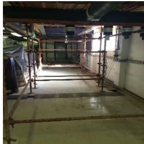
Figure 4: LaDepa region with scaffloding underneath the finished slab.
