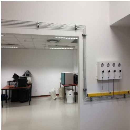
Figure 3.1: Gas lines and regulators installed in the laboratory.
