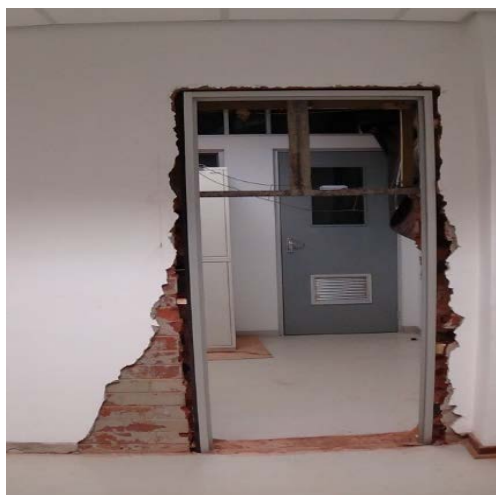
Figure 1: Frame fitted after breaking the wall view 1.
