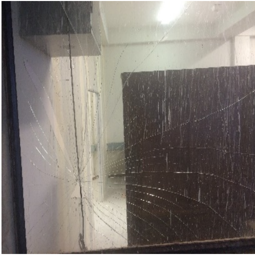
Figure 1: Damaged window between lab and office arera.
