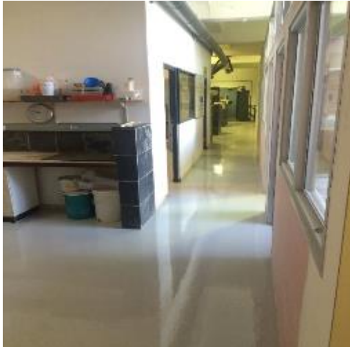
Figure 1: Laboratory Floors refurbished with epoxy coating.
