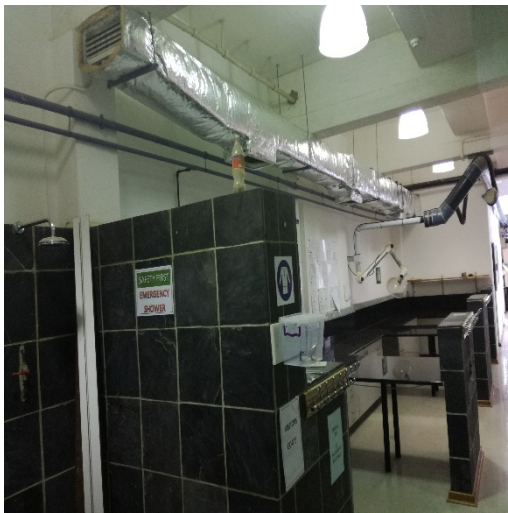
Figure 3.1: Air duct insulation.
