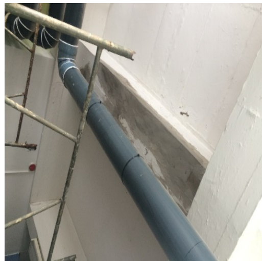
Figure 4: Beam spalding repaired
