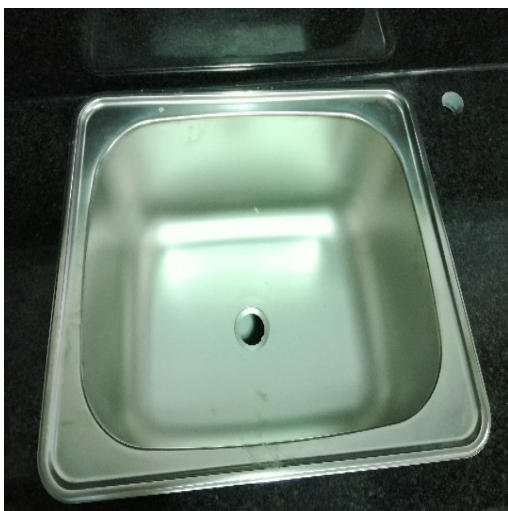
Figure 4: Sinks not fitting properly in granite tops.
