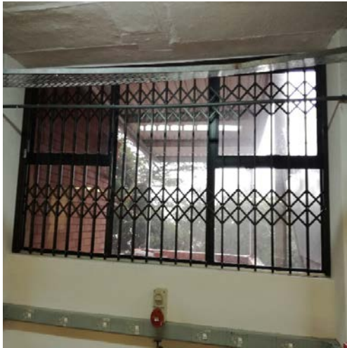
Figure 1: Window burglar guards installed.
