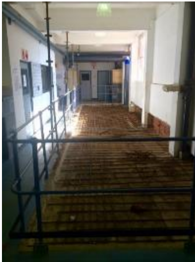
Figure 1: Basement 1 slab foundation with metal reinforcement grid.
