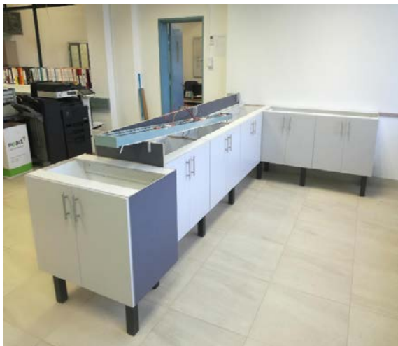
Figure 3: Trunking to be fitted on kitchen counters
