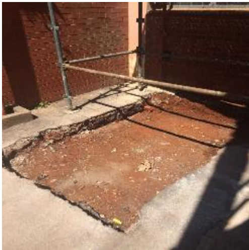
Figure 3: Concrete removed for the wash basin area.
