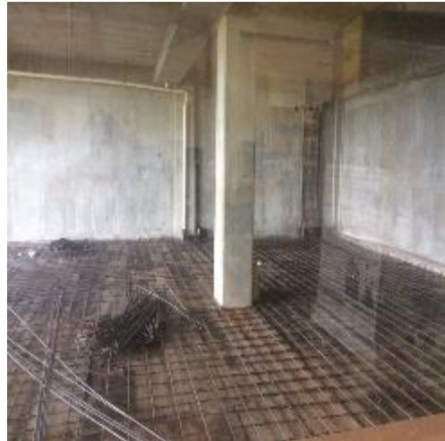
Figure 4: New slab foundation with grid layer (underpinning).
