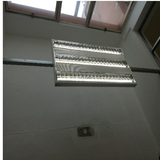
Figure 3.2: New lights fitted in partitions
