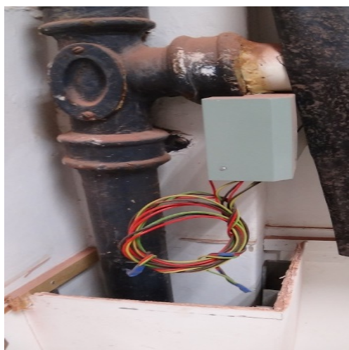
Figure 3: Trunking wire exposed.
