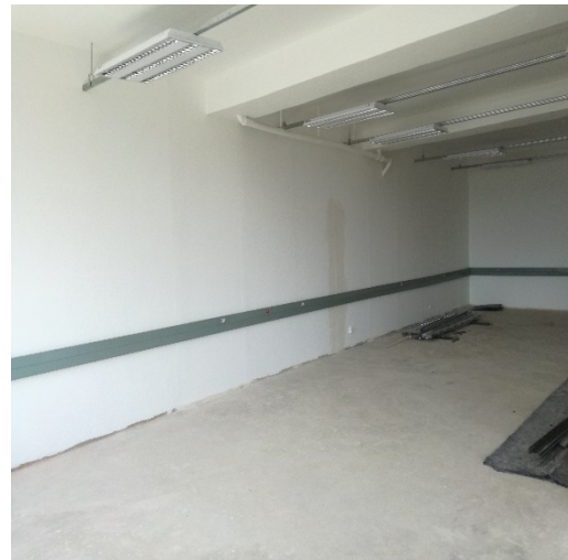
Figure 3.2: New lights and trunking fitted on the new office area.
