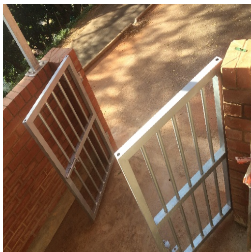
Figure 4.2: Problem encountered with the narrow gates fitted for the wash area.
