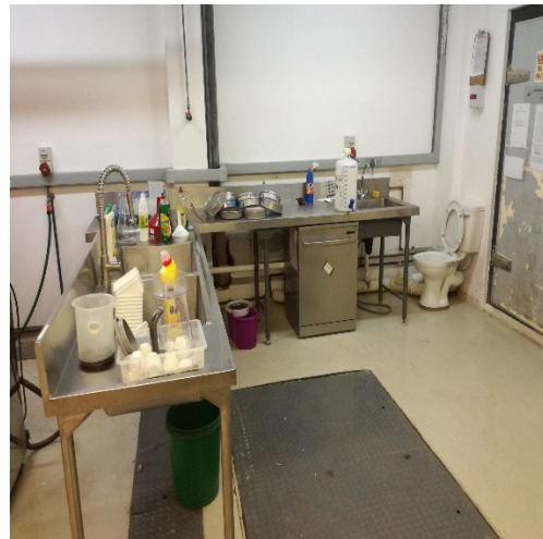
Figure 3.2: Sink positioned and plumbing done.
