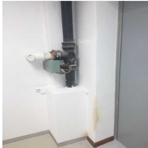
Figure 2: Exposed trunking wires.
