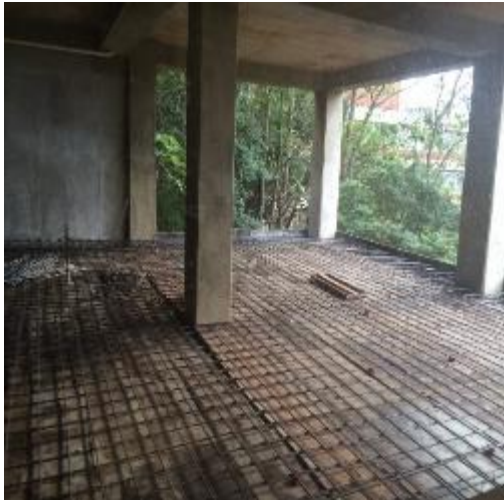
Figure 3: New slab foundation with grid layer (underpinning).
