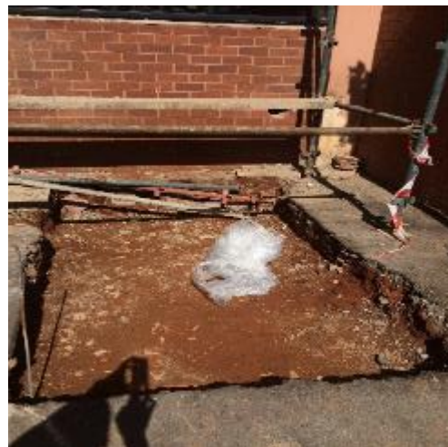
Figure 4: Tar concrete removed from the wash station.
