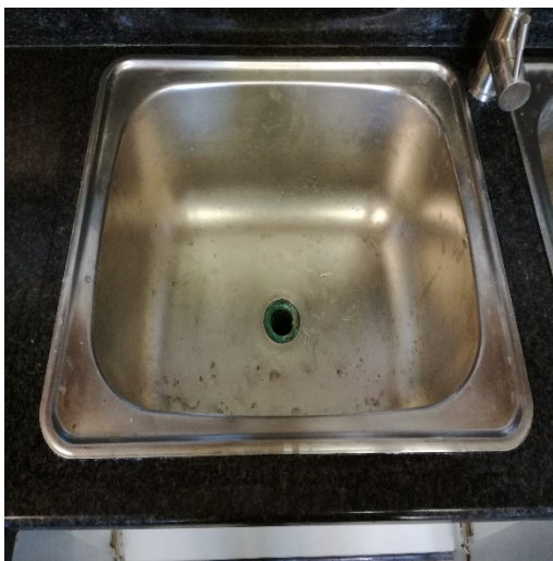
Figure 4.1: Sinks fitted properly after granite adjustment.
