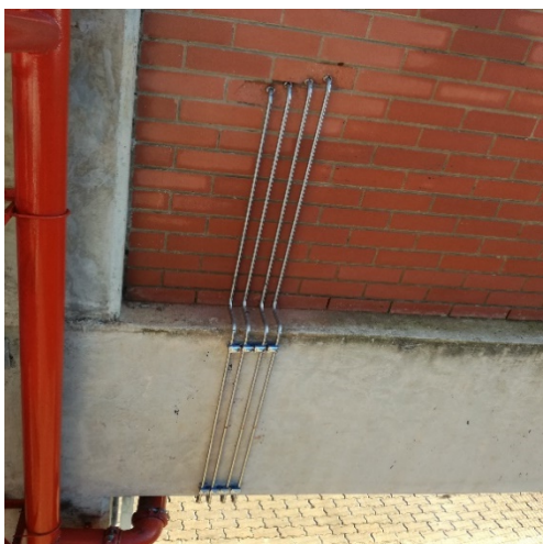
Figure 3.3: Gas lines going into the gas cylinders from the lab.
