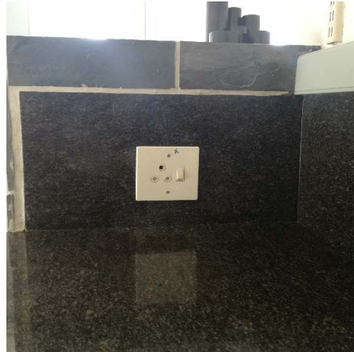
Figure 2: Plug points fitted into the granite.
