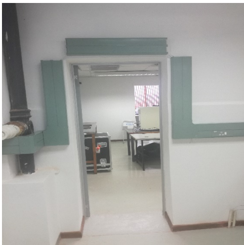
Figure 5: Fitting of the trunking in chemistry room.
