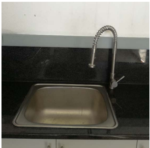
Figure 4.2: Taps fitted.
