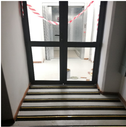
Figure 1: Non-slip tracks fitted on ramp.
