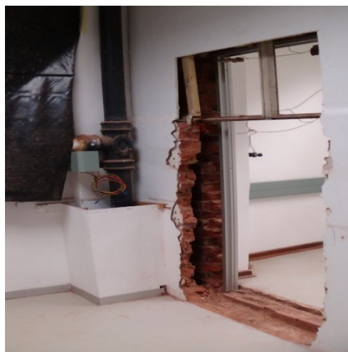
Figure 2: Frame fitted after breaking the wall view 2.
