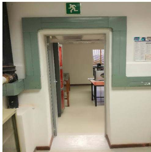
Figure 6: Completed trunking in chemistry room.
