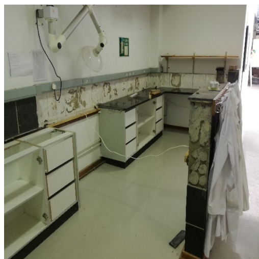
Figure 5: Cracked granite removed .
