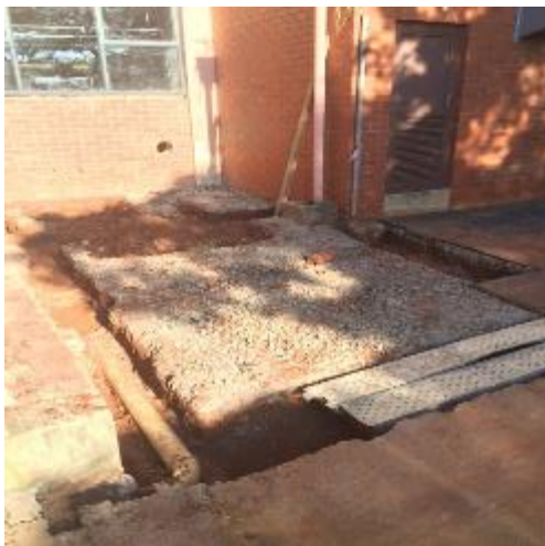
Figure 3: Wash station foundation preparation.
