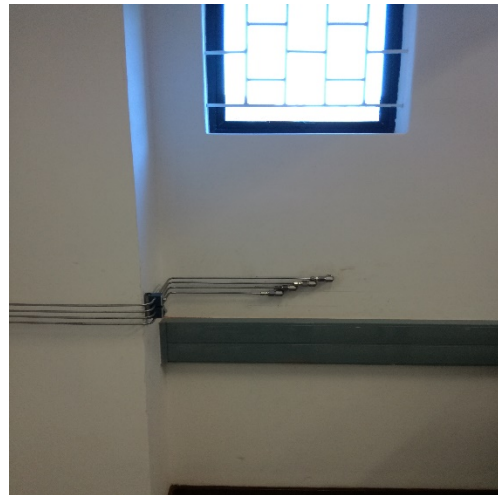
Figure 3.2: gas lines going through the wall.
