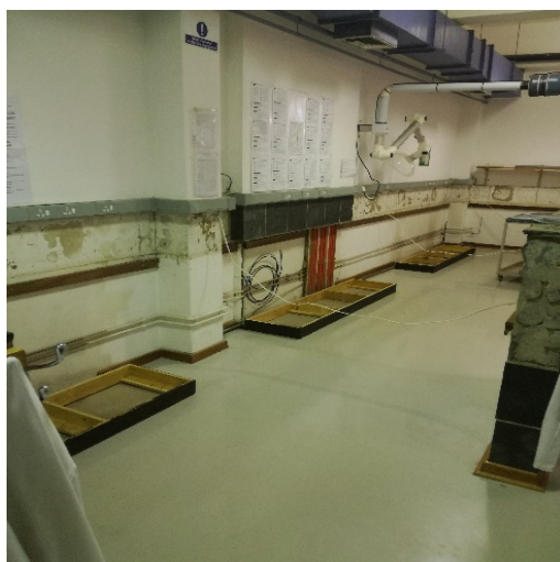
Figure 4.1: Installation of bases for the cupboards.
