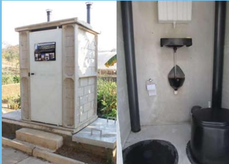
soak-away. Installation of urine diversion toilets was part of the municipality's overall strategy to provide sanitation for all citizens. These toilets were chosen because providing a pipe network and a treatment system would have been prohibitively expensive and impractical due to the hilly landscape. To date, about 85 000 urine diversion toilets have been installed in eThekweni.
